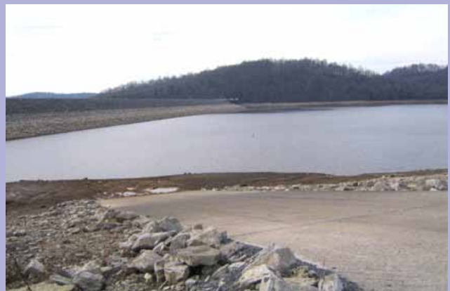
During last year's drought, water levels in Normandy Reservoir dropped so low that boat ramps no longer reached the water.
